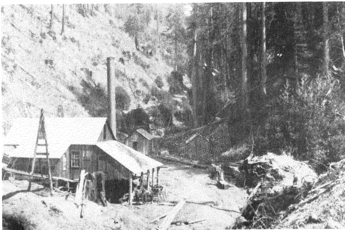
"Shingle King" Purdy Pharis turned out 70,000 shingles a day in the 1880s from this shingle mill in Purisima Canyon. One of the few innovators in Peninsula lumbering, he invented machinery for making shingles.
